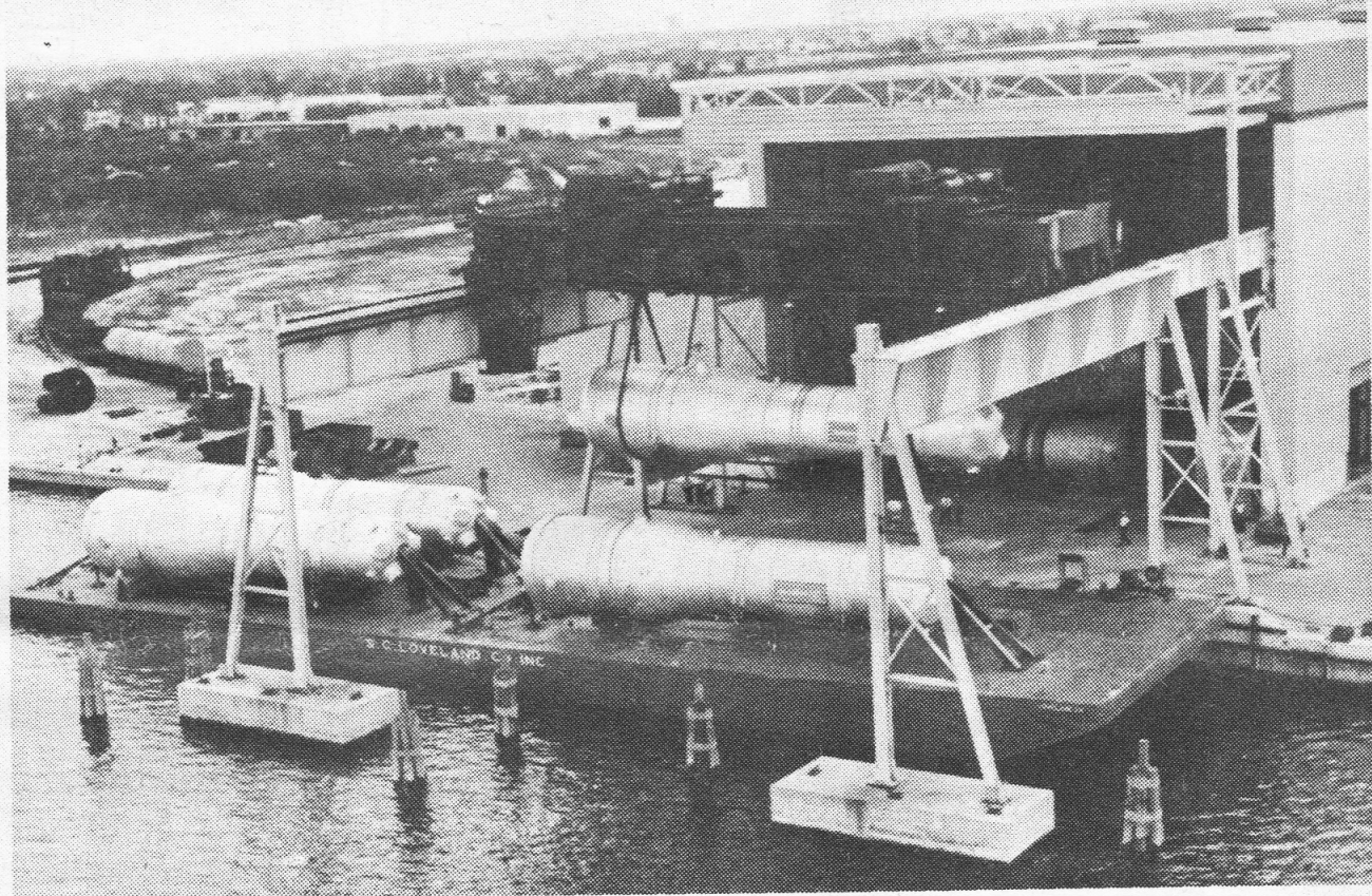
CALIFORNIA BOUND -- Four huge steam generators, representing one of the heaviest shipments ever made on a single barge, are enroute from Tampa, Florida to Pacific Gas and Electric Company's nuclear power plant project at Diablo Canyon in San Luis Obispo County. The shipment weighs more than 1,480 tons and is scheduled to arrive at a special barge landing facility near Avila Beach this week. The steam generators, each of which is 68 feet long and 14 feet in diameter, were manufactured by the Westinghouse Electric Corporation. They are an integral part of the 1,060,000-kilowatt nuclear fueled electric generating unit now under construction and scheduled for early 1973 commercial operation.
